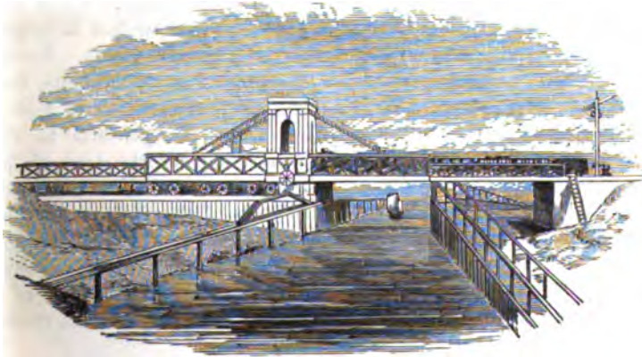
DRAW-BRIDGE OVER THE ARUN.
